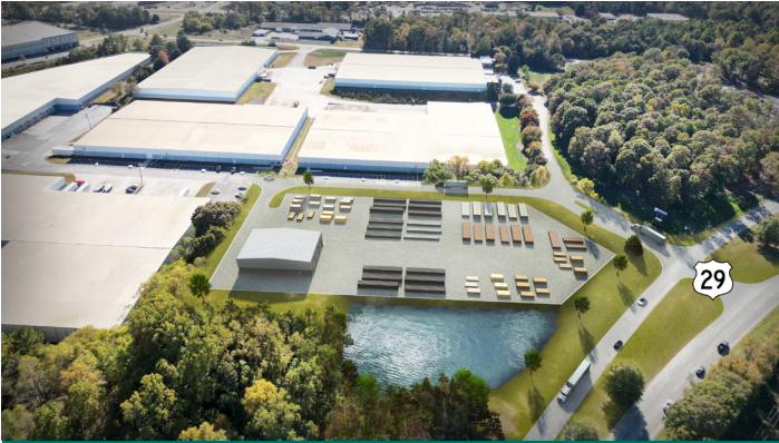
Equipment storage with 2,500 - 12,000 SF Build to Suit Shop / Warehouse
