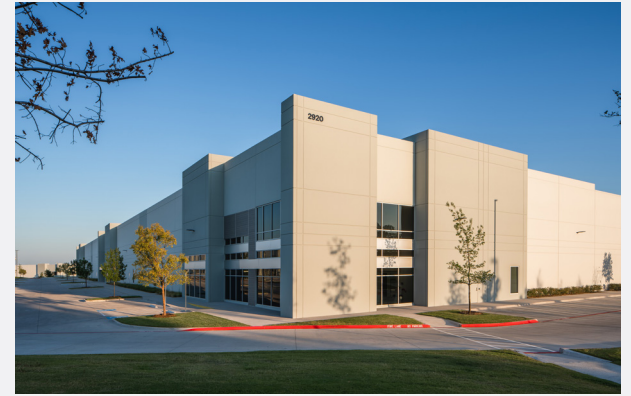
// PARC NORTHEAST RICHARDSON, TEXAS
