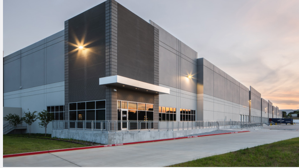
// PARC SOUTHWEST IRVING, TEXAS
